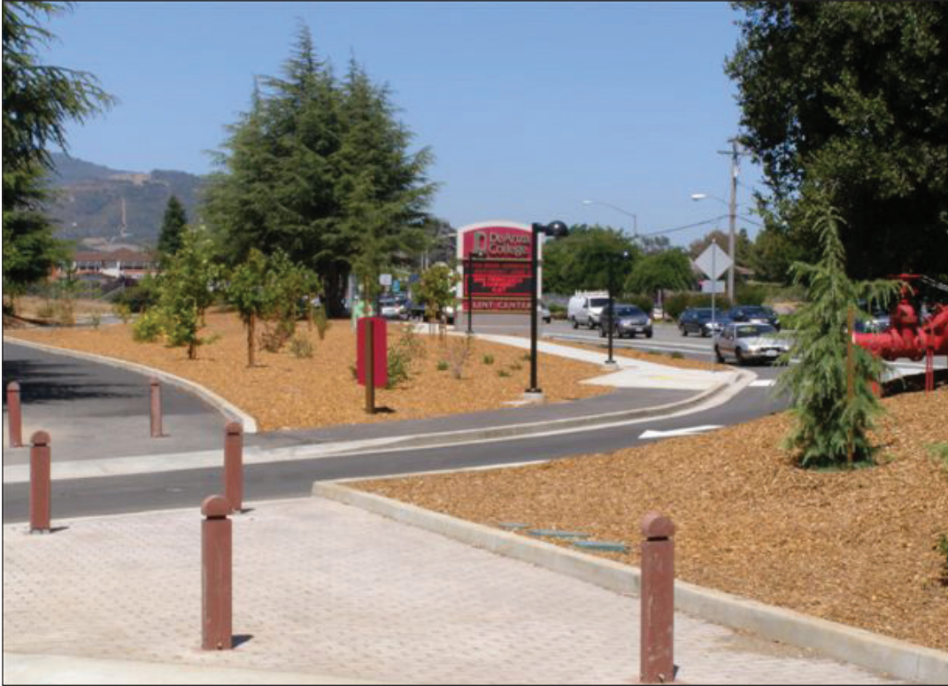
New campus entry adjacent to Flint Parking Structure
